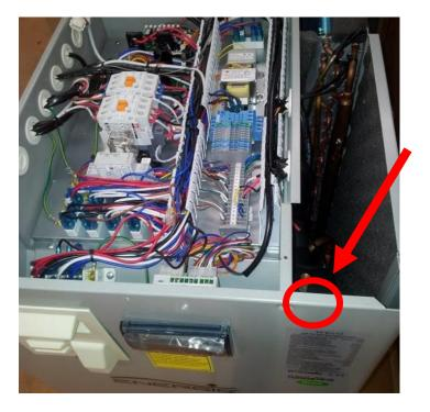
The installer should make the purge on this air vent until reach a small water trickle.
